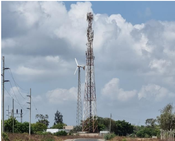
Plate 4-6: A communication mast noted within the project area
