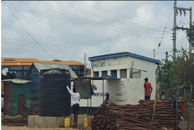
Plate 4-12: Storage tank at the Public Toilet supplied by a water bowser sourcing water from Hindi area
