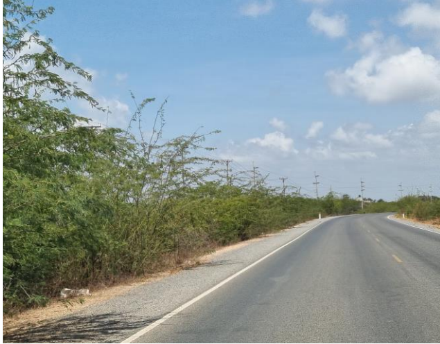
Plate 4-7: : Prosopis Juliflora along the main Mombasa-Lamu road an indication of using contaminated materials
