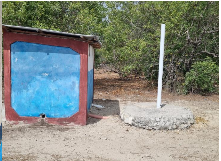
Plate 4-17: One of the Soak Pits constructed adjacent to the Toilet
