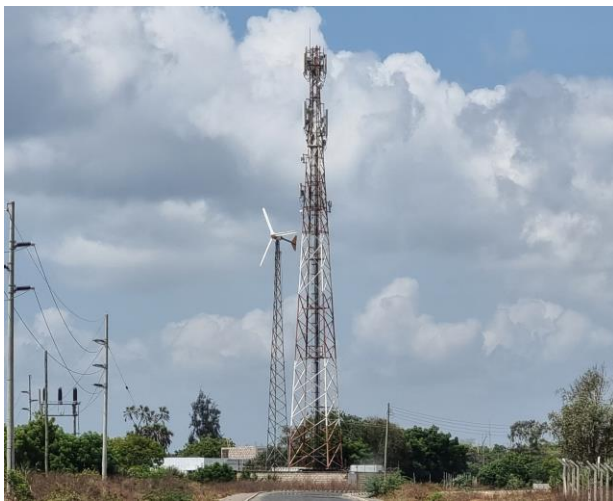
Plate 4-9: A communication mast noted within the project area
