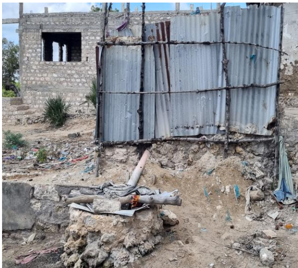
Plate 4-18: Makeshift Toilet connected a soak pit
