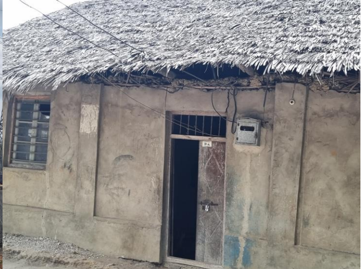
Plate 4-21: Power Connected to one of the residential Homesteads at Mokowe area
