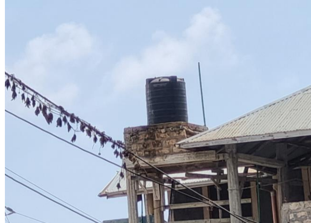
Plate 4-14: Water storage at one of the roof tops that was reported to be pumped from shallow wells
