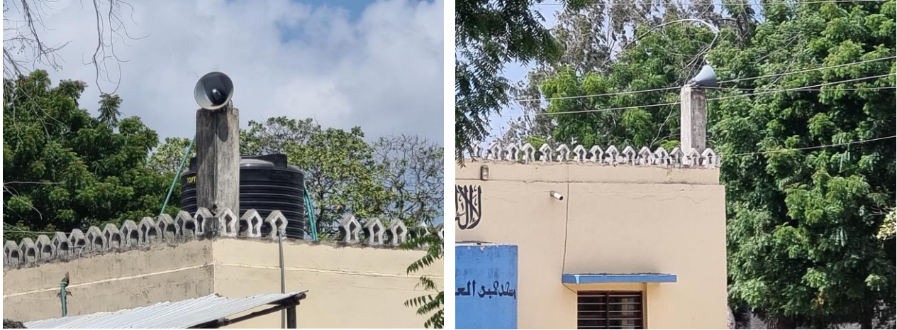
Plate 4-6: One of the Public Address systems noted in the area
